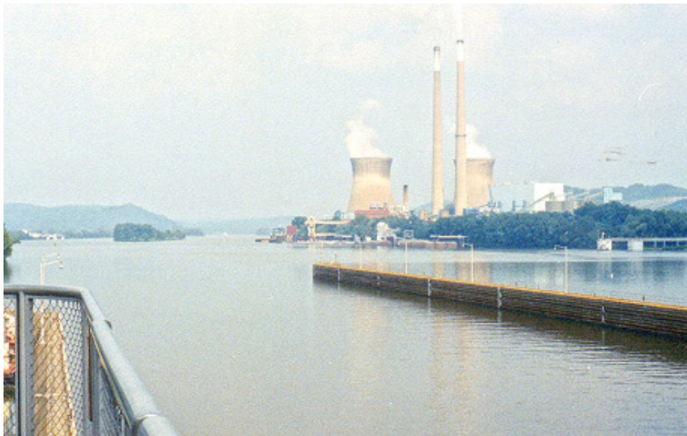
Pleasants Power Station is a coal-fired plant in West Virginia.
